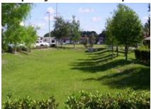
Example of a properly maintained dry stormwater pond; vegetation is properly mowed to the correct height and is free of debris.
