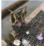
Example of an improperly maintained stormwater pond. Vegetation and trash have accumulated and clogged the grate which prevents the flow of water.
